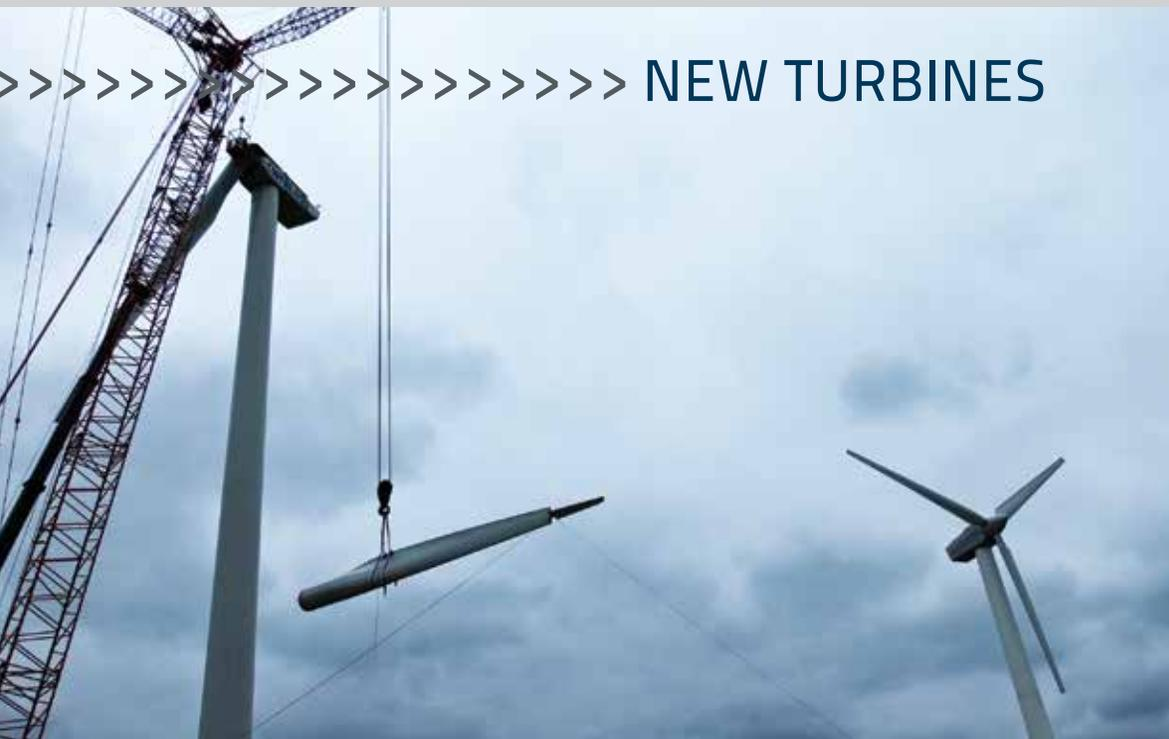
Case Western Reserve's Wind Energy Research & Commercialization Center (WERC) added two new turbines—a Vestas V-27 225-kilowatt turbine and a utility-scale Nordex N-54 1-megawatt turbine—to be used as platforms for the development of wind power supply chain products and long-term educational and training opportunities.
